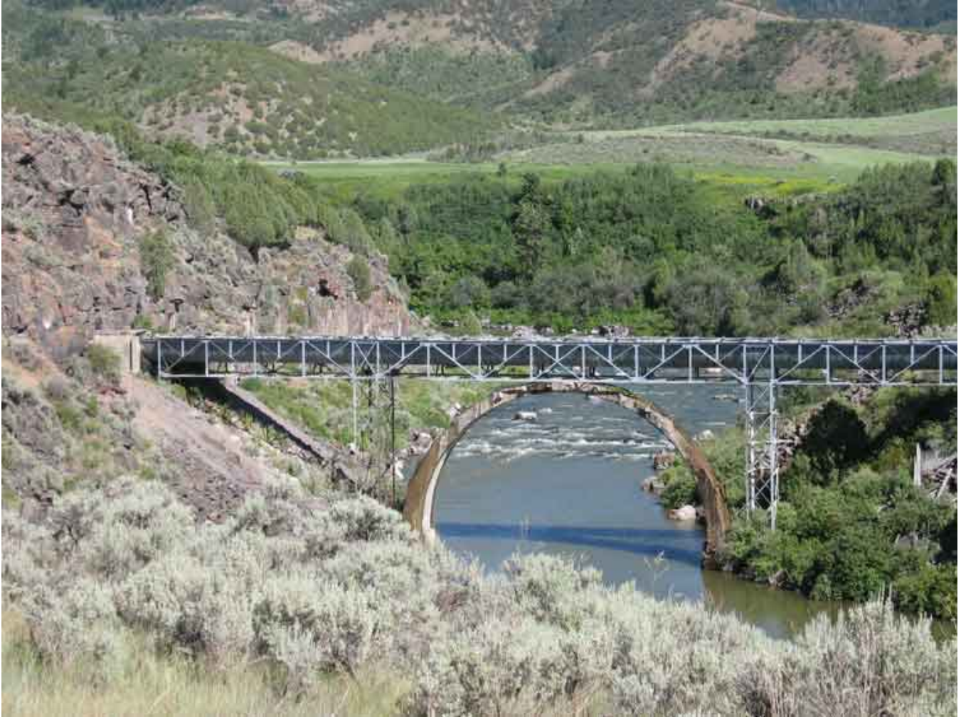
Part of the Last Chance Canal system a mile north-east of Grace. Water is diverted from the Bear River to the canal at a dam another mile or so upriver to the left of photo.
