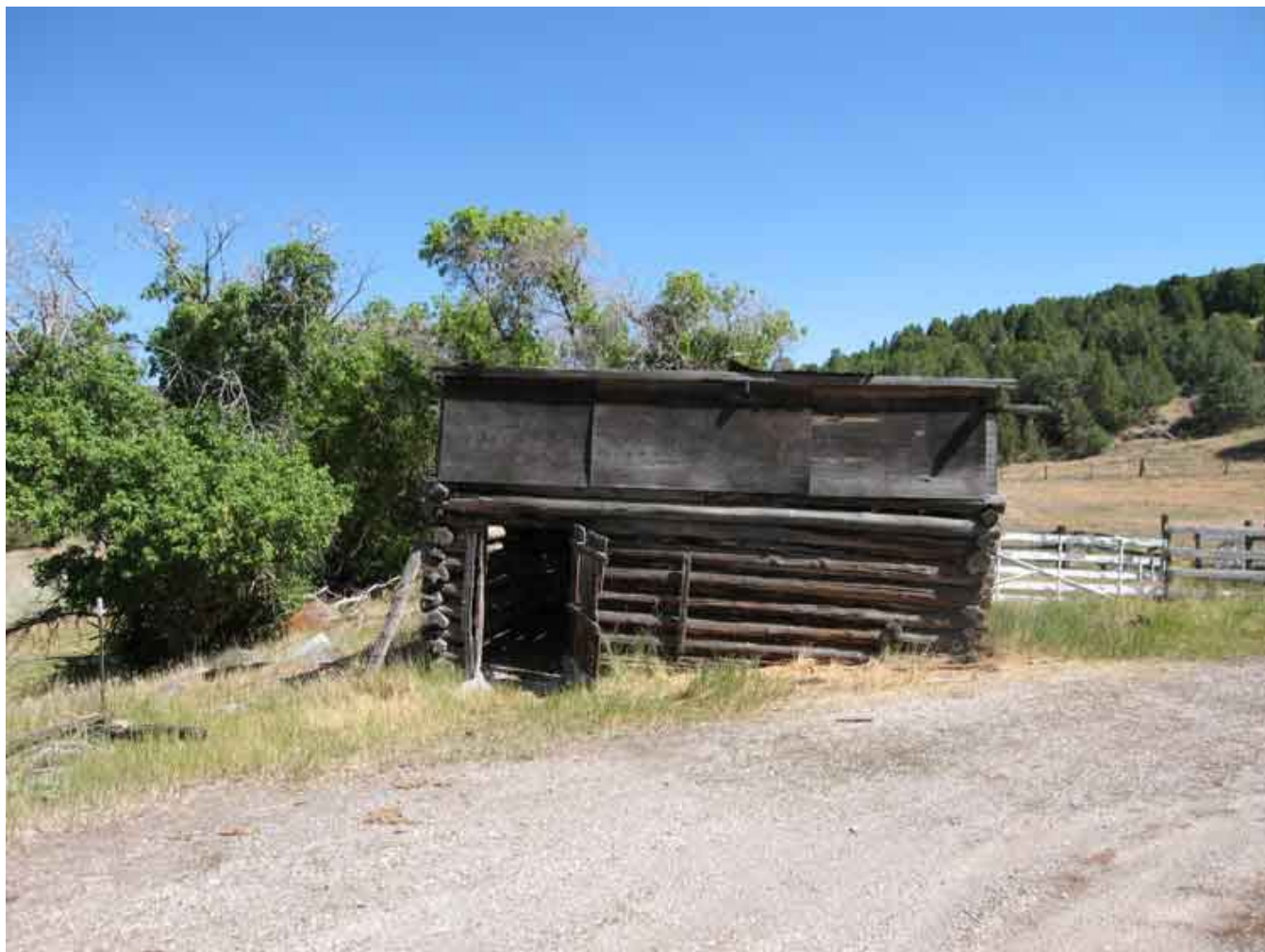
Closer view of the old barn. The roof has apparently been improved upon over the years but the side logs appear original.
